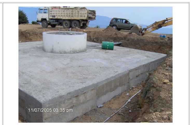
FOUNDATION OF SIDIROCASTRO WIND FARM
