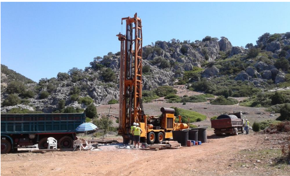
VIEW OF THE EXECUTION OF THE OPEN HOLES AT THE SUBSTATION AREA OF “DESFINA” WIND-FARM FOKIDA PREFECTURE
