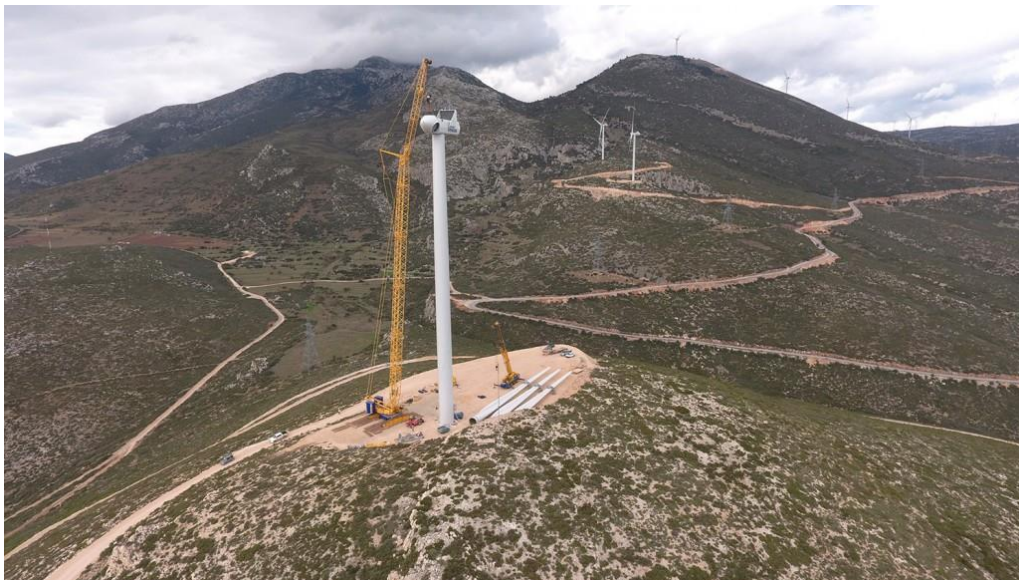
VIEW OF THE CONSTRUCTION OF “PEFKIAS” WIND-FARM VIOTIA PREFECTURE
