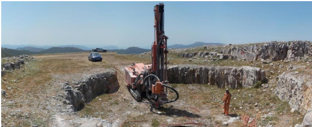
VIEW OF THE INVESTIGATIONS EXECUTED AT THE WIND TURBINES BASE AREAS AT THE MOUNTAIN RIDGE WHERE THE “GROPES – RACHI GKIONI” WIND-FARM IS TO BE CONSTRUCTED LAKONIA, PELOPONNESE PREFECTURE
