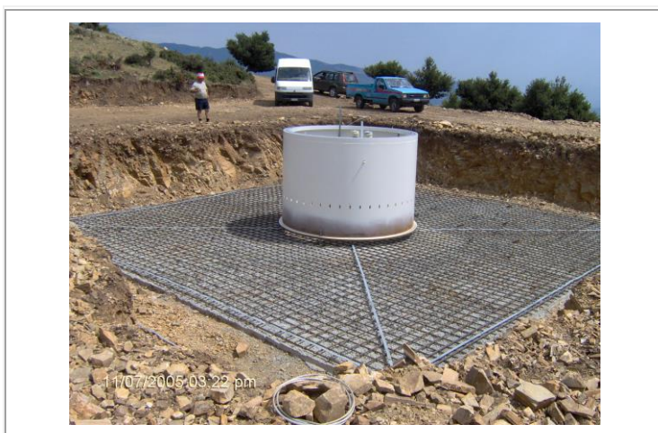
FOUNDATION OF SIDIROCASTRO WIND FARM
