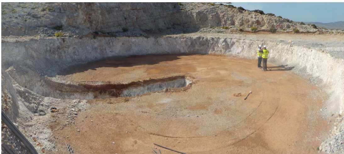
VIEW OF INVESTIGATIONS FOR THE QUALITY CONTROL OF BACKFILL LAYER AT WIND TURBINES BASE AREA LAKONIA PREFECTURE
