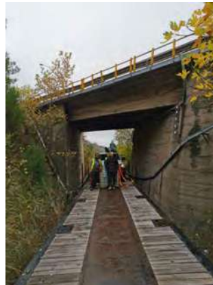
Railway Line Drilling
